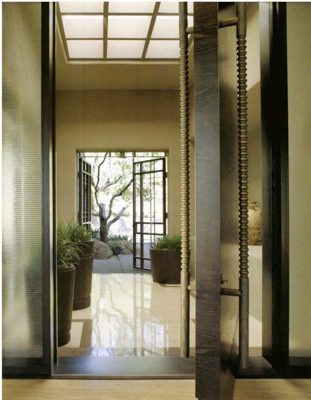
STEELY EXPRESSION The foyer, with a cubed skylight, leads to a steel gate original to the house. Interior designer David Michael Miller implemented the center-pivot door in the foreground a couple of years before the major remodel; it comprises ebonized white oak, an embossed bronze plate and bronze poles cast by Corbin Bronze in Kansas City, Kansas.
